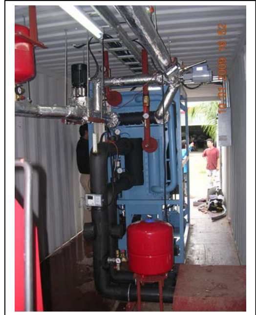
10 RT (35 kW) Automatic Hot Water Operated Chiller from Thermax
