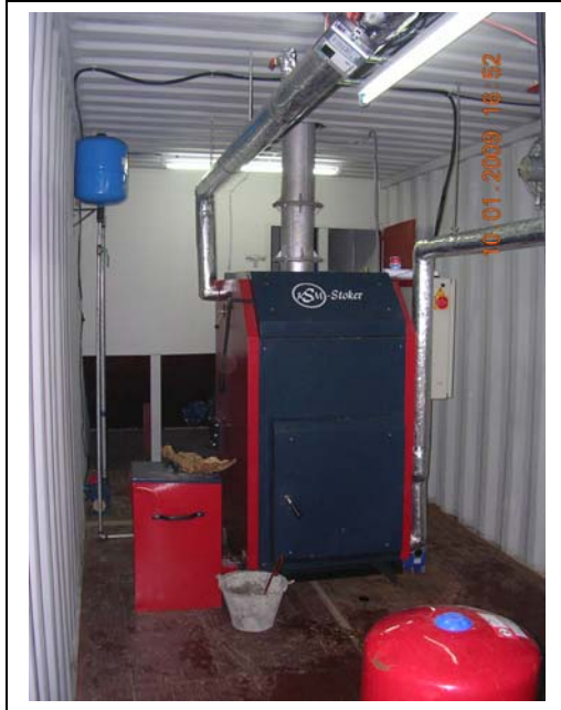
50 kW Automatic Biomass Boiler from KSM-Stoker
