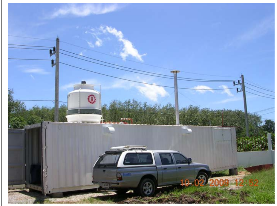
Containerized Biomass fuelled 10 RT Absorption Chiller
