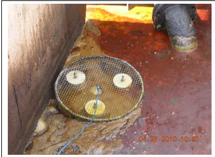
In the morning of April 25 most of the old dark oil had been removed, and more CPO like oil covered the surface of the pit. It is believed that POME running into the pit is mainly coming from the canal collecting POME from underneath and around the sterilizers. The canal outlet to the pit is seen in the top center of the picture.
