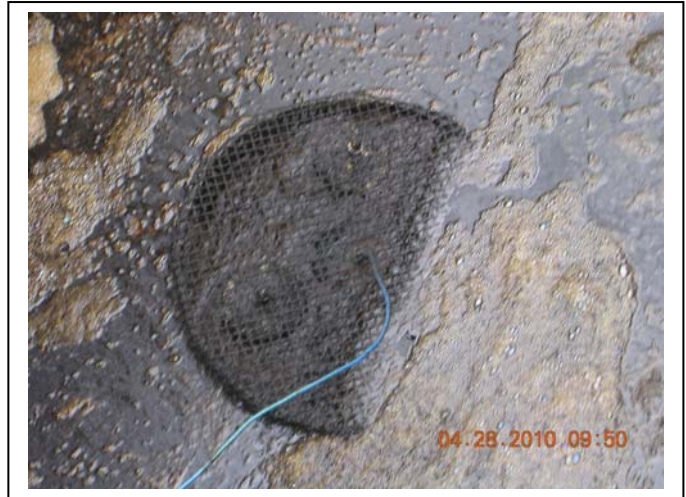
Close up of the oil skimmer; note all the black fiber on the skimmer
