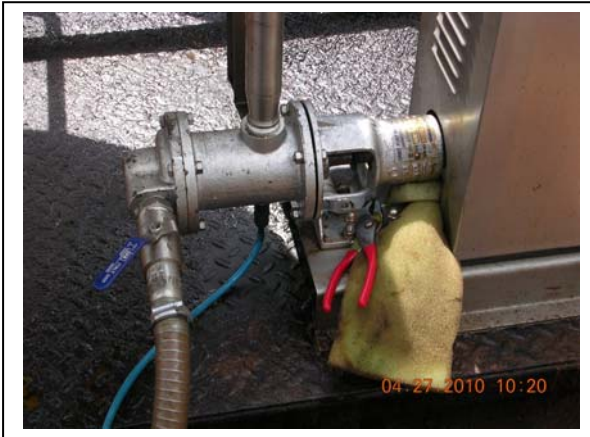
Inaccuracy in the sampling of POME from the pit, resulted in the mounting of a sampling valve and a small hose at the test unit pump (outlet was higher than inlet)
